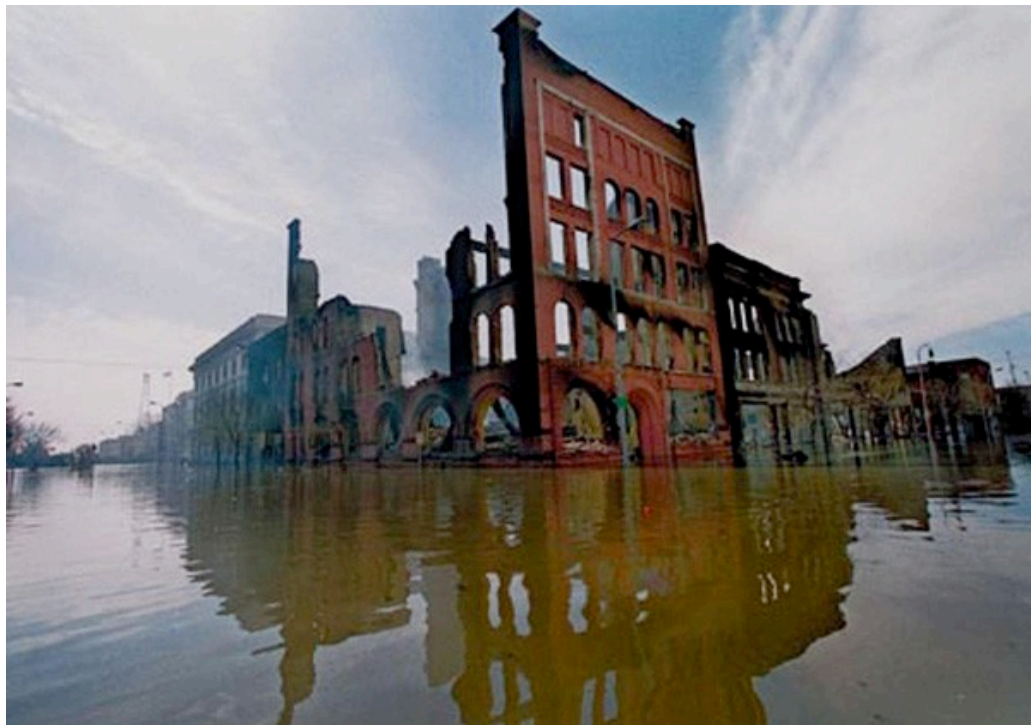
Downtown Grand Forks, North Dakota, 1997, after floodwaters ruptured a gas line, igniting a fire that claimed eleven office buildings. Photo by Eric Hylden, Grand Forks Herald .
